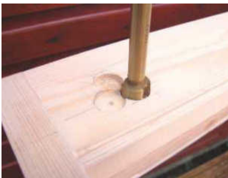
STEP 14. Set out the trefoils if required. Cramp an offcut underneath the apron and bore holes using the drill stand
